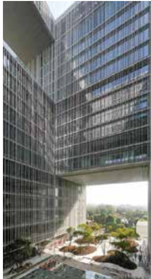
<5층 Roof Garden>
